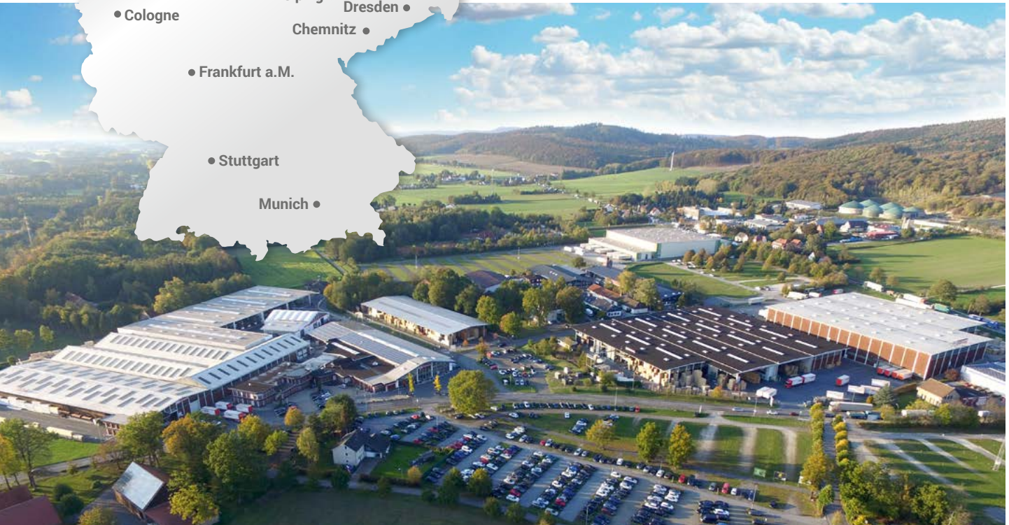
Production site Halle/Westfalen, Germany
